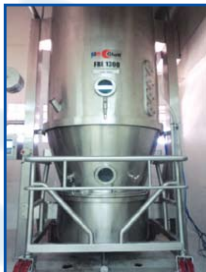
The newly installed FBE 1300 fluid bed equipment at Regal Pharmaceuticals Ltd
